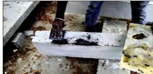
Figure 4 Application of Putty
