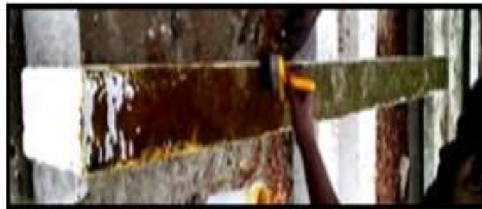
Figure 5 Application of Epoxy Resin
