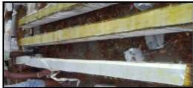
Figure 6 CFRP Retrofitted Beams
