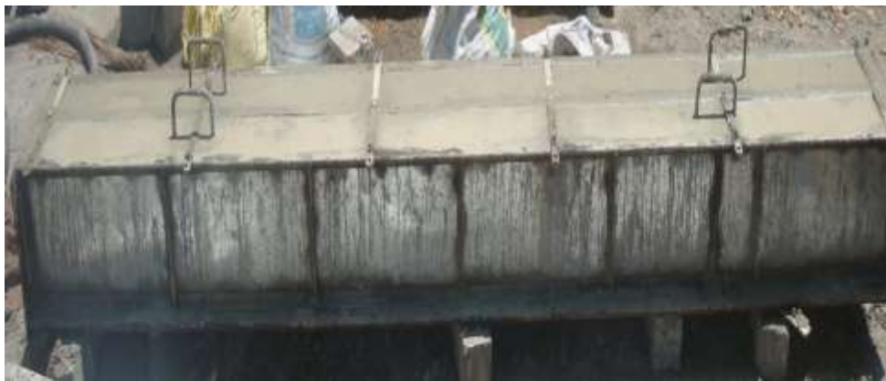
Figure 1 Casting of Beams
